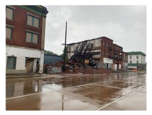
August 11, 2023, the structure located at 1006-1008 S 4th St collapsed causing damage to the adjoining structures on the 1000 Block of S 4<sup>th</sup> St. A structure engineer viewed the structures and recommended that all the buildings be demolished immediately due to danger of possible
