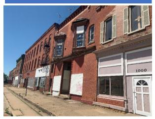
further collapse. Late August 2023 the structures from 1000 to 1008 were demolished. Given these contained regulated asbestos containing material (ACM) a tarp was placed over the ACM debris and will be disposed of as friable ACM at a landfill.
